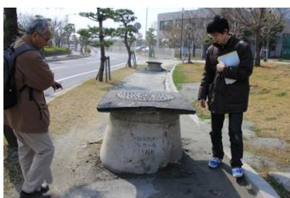
**Fig. 2** Raised manholes caused by soil liquefaction (Urayasu City).
