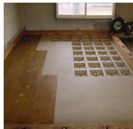
Figure 3. High sound insulation double floor structure.
